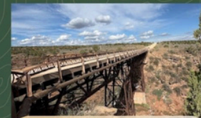
Querino Canyon Bridge
